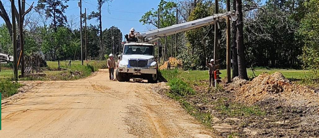
Lowndes County: Utility crews have started moving lines on the Coleman Road NW paving project in Hahira.
